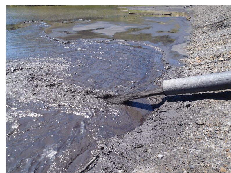
Figure 1. Fine coal refuse slurry at discharge pipe
